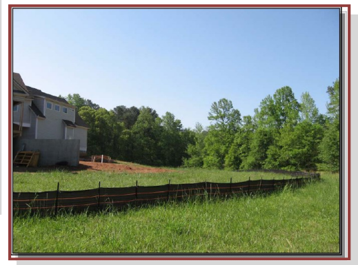
Example of Good Erosion Control
