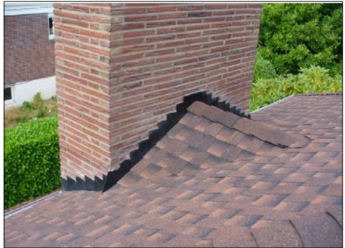
Cricket or saddle at chimney
