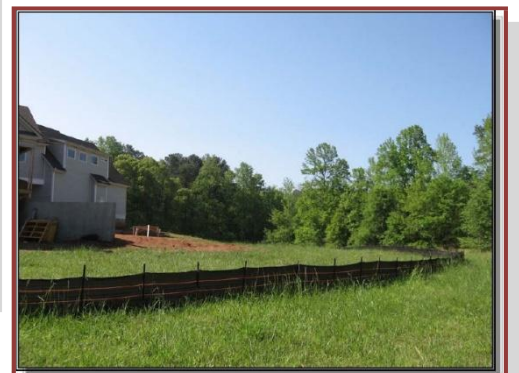
Example of Good Erosion Control
