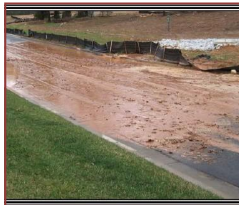
Example of Poor Erosion Control
