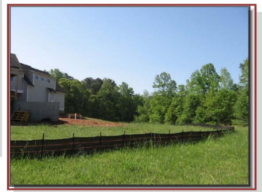
Example of Good Erosion Control
