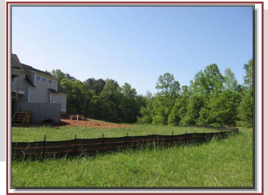
Example of Good Erosion Control
